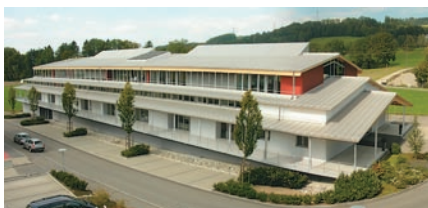
Our international facility in Schenkon, Switzerland
